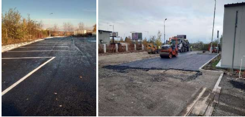
Figure 1 Construction of demonstration unit with bottom ash
