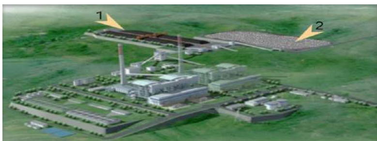
Figure 1 Spatial location in the area of the thermal power plant for the accommodation of coal (1) and FGD gypsum (2)
