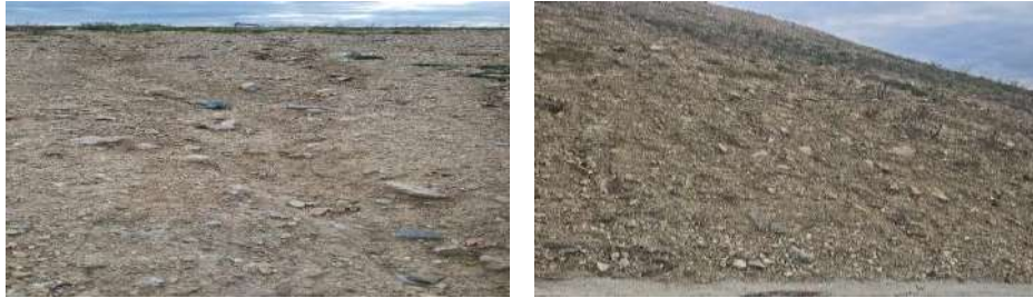
Figure 6 Erosion on the landfill before bio stabilized material is used
