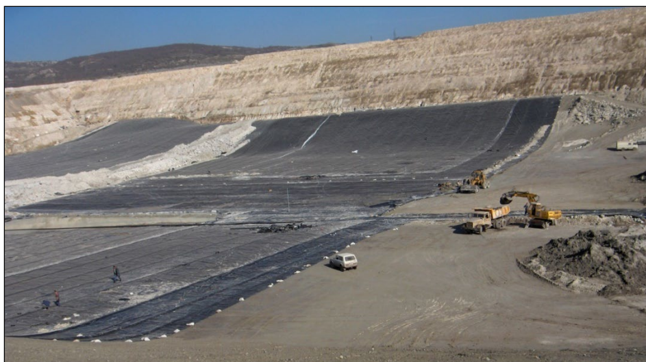
Figure 2. Placing the waterproofing foil on the bottom of the cassette 2
