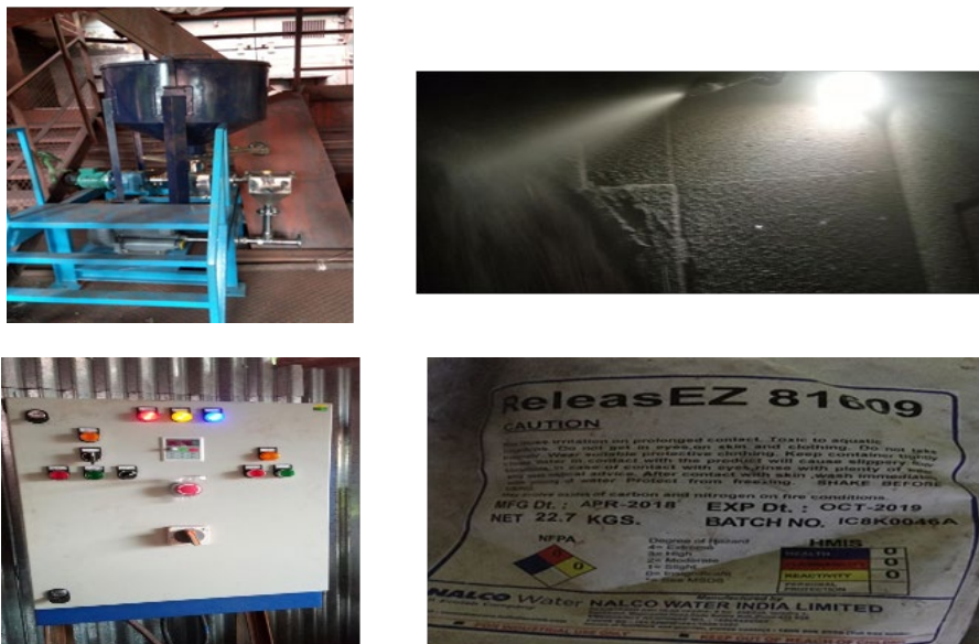
Figure 7. Chemical Dosing System and Dosing Points
